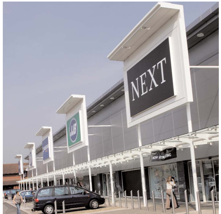
Maybird Retail Park, Stratford-upon-Avon, showing refurbished frontages.
